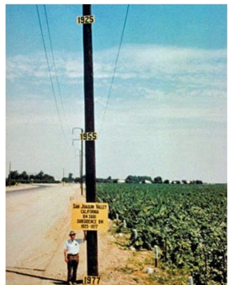
Figure 18. Fifty years of subsidence (over 20 feet) in California’s San Joaquin Valley. Image courtesy of National Geodetic Survey (NGS).
